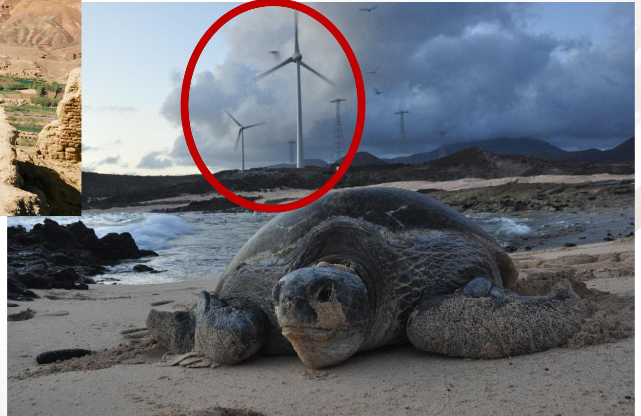
Ascension Island Five, 330kVA wind energy convertors (2010)
